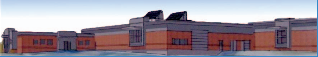
The reconstructed Muriel P. Frye Building, site of the KVCC Energy Services and Technology Center.
